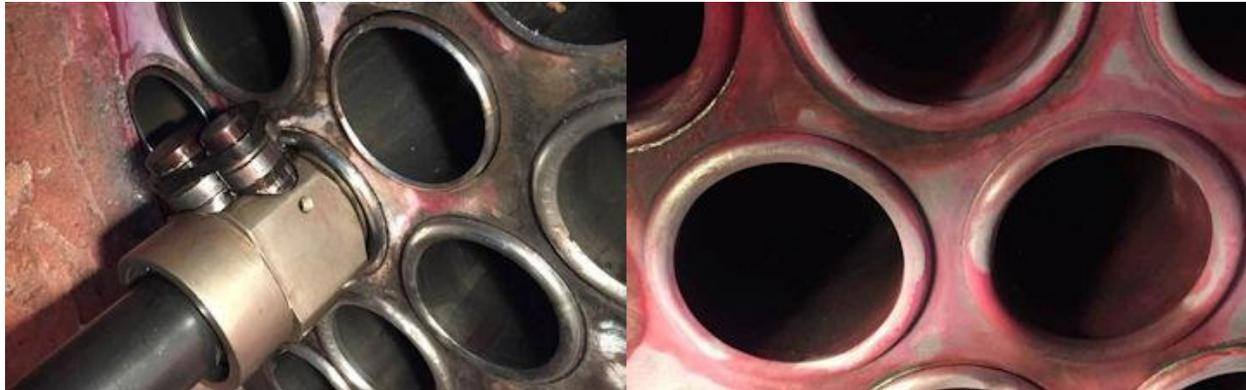
We bead tubes for one reason, to transfer the heat from the tube end into the tube sheet. If not burn back and cracking can occur therefore with a fully beaded tube end the heat from the gases transfer into the tube sheet.
